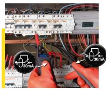
By simultaneously pressing the double command, you can cause a fault current sufficient to trip the RCD to flow through a low-impedance load.
