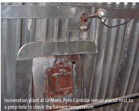
Incineration plant at Le Mans. Pyro-Contrôle sensor placed next to a peep hole to check the furnace temperature.
