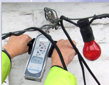
Pull test on anchorage points
